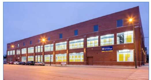
Uncle Bob's Self Storage recently opened this converted facility at 1625 S. Ashland Ave., Chicago, IL
